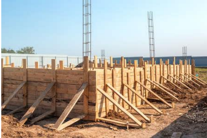
Timber formwork.
