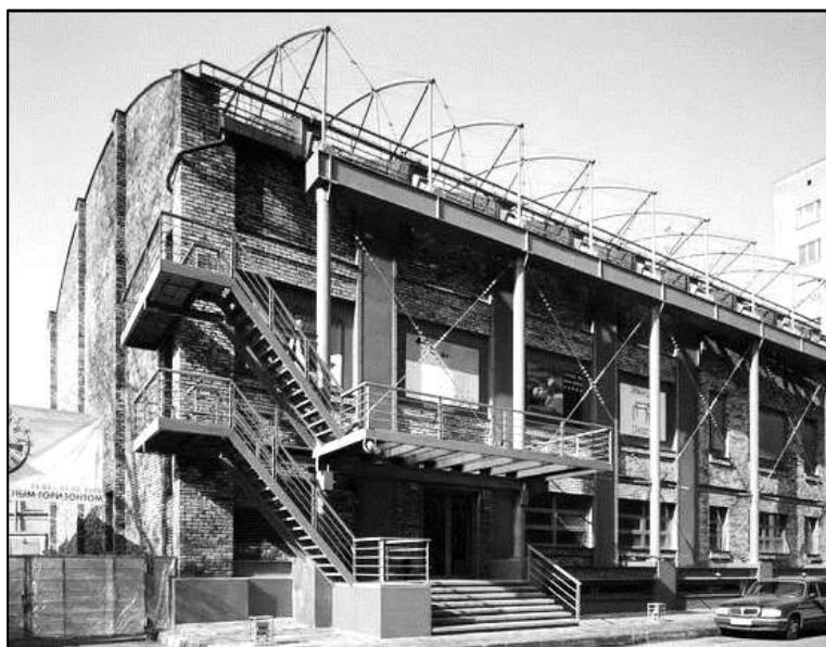
Former factory on Zoologicheskaya Road
