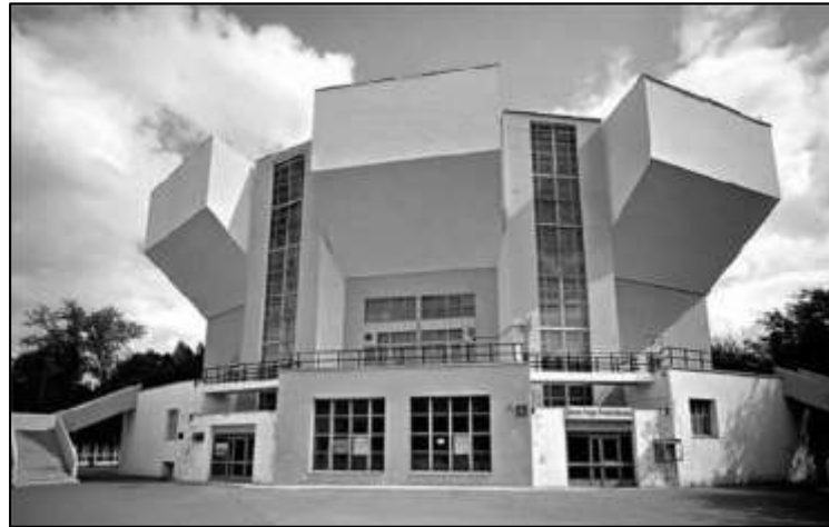
Constructivism – Club by Rusakov (arch. K.S.Melnikov)
